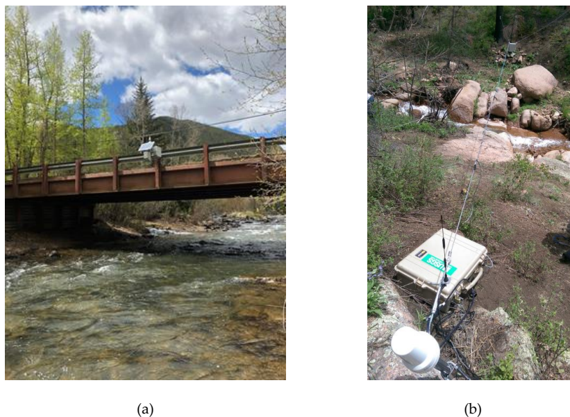
Figure 3. Photographs of typical radar deployments from (a) bridge along Clear Creek near Lawson, Colorado, and (b) cable stays in Waldo Canyon, Colorado, USA.
